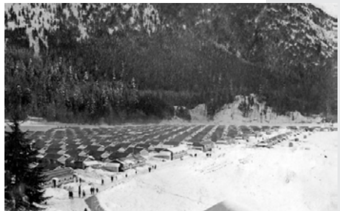
Above: Snowy row houses looking east and north, 1943. NNM 2012.45.1.12
